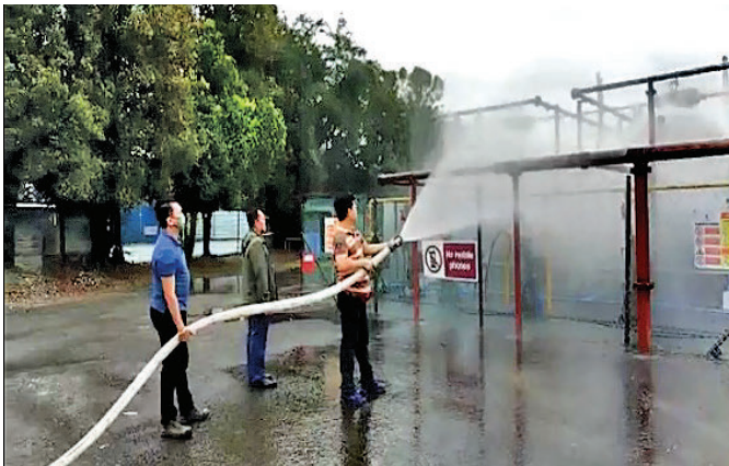
Fire Hydrant Testing and Training
